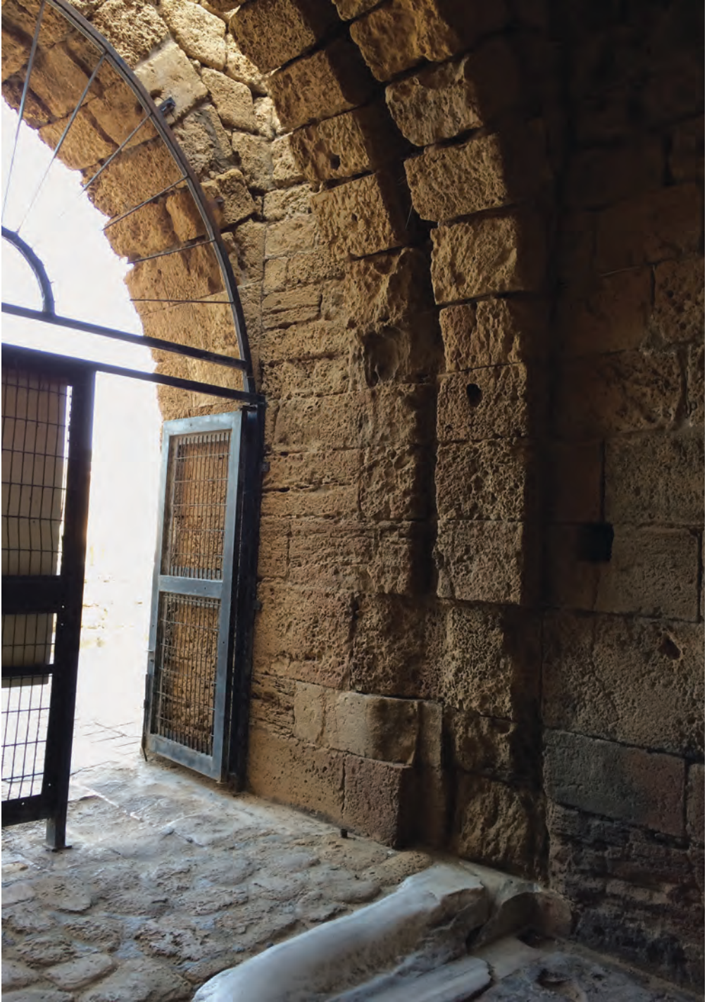
Caesarea, outer gate of the eastern gateway, featuring a slot machicolation, portcullis groove, lower socket for a leaf door and pocket in the wall for a locking bar. ( Michael Fulton )
